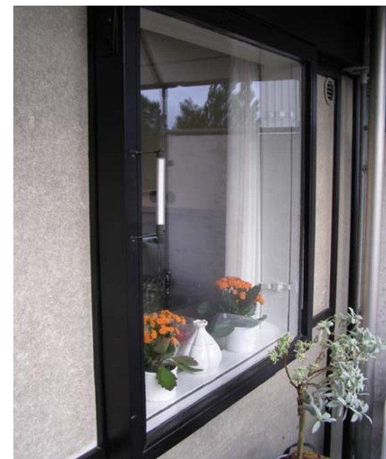
Skydevindue mod altangang.
